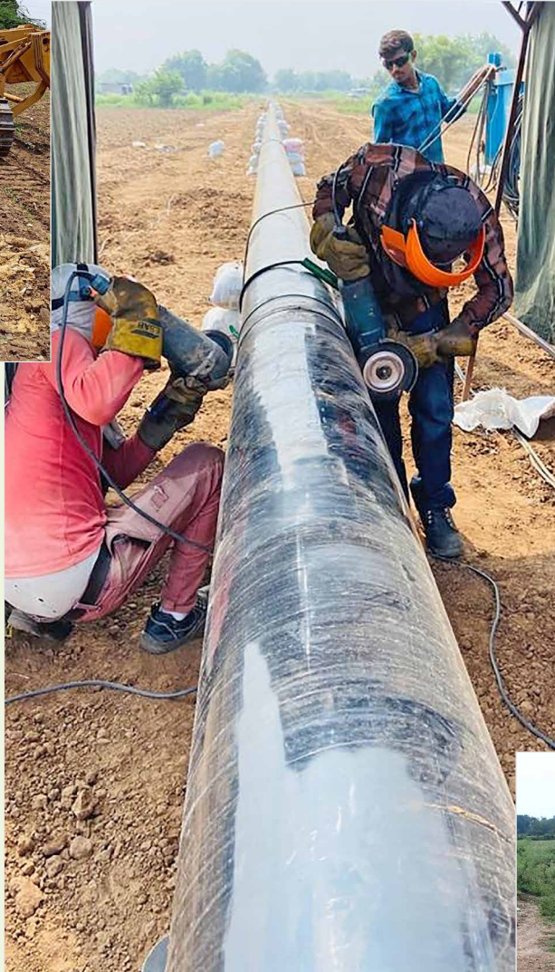
Welding and Interpass Burfing at Ch 316 Group 4 (M/S AIPL)
