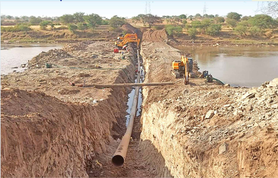
Submerge crossing at Anas river (Group-08)
