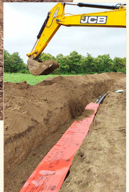
Backfilling in group-09 ▶
