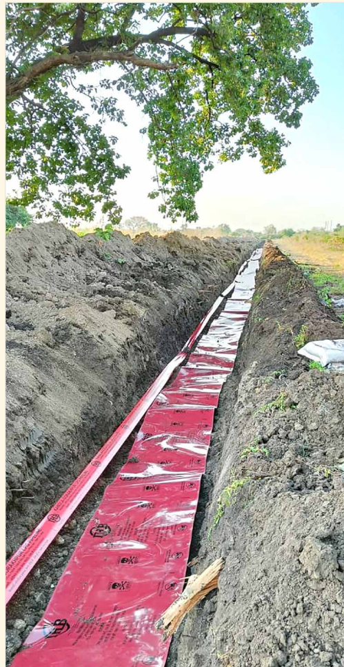
◀ Backfilling with Warning Mats
