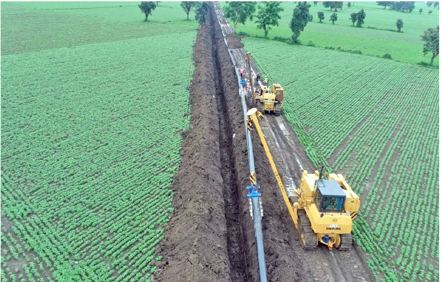
Pipeline lowering in MP ▲
