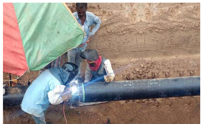
Welding work under progress in UP
