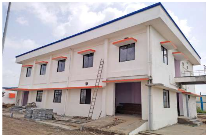
Workshop building Dumad
