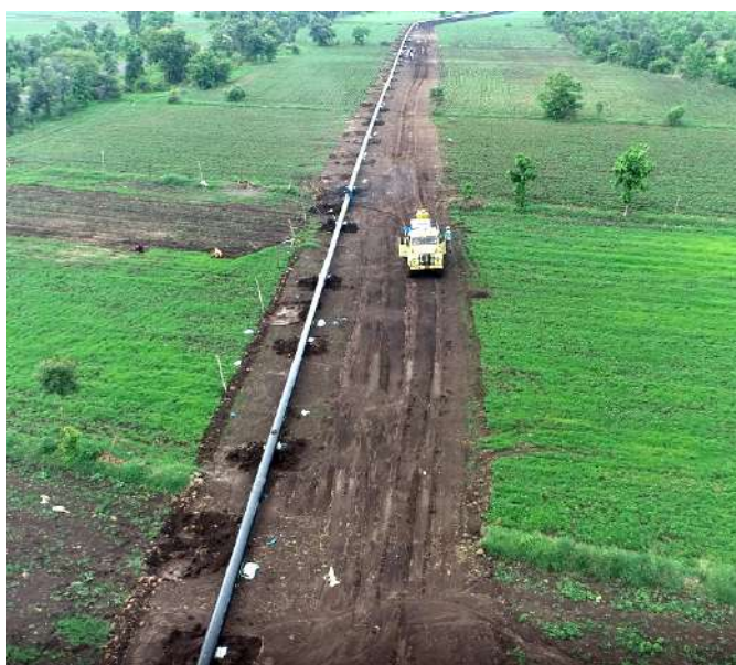
Welded string in MP
