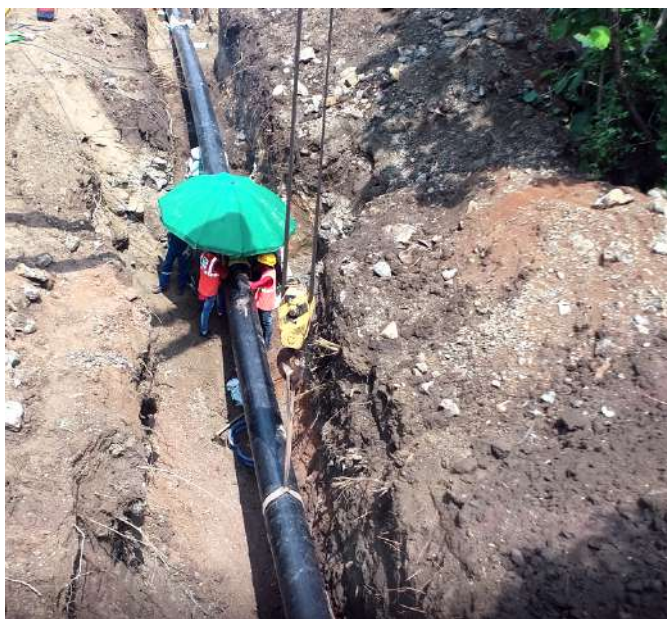
Tie in MP
