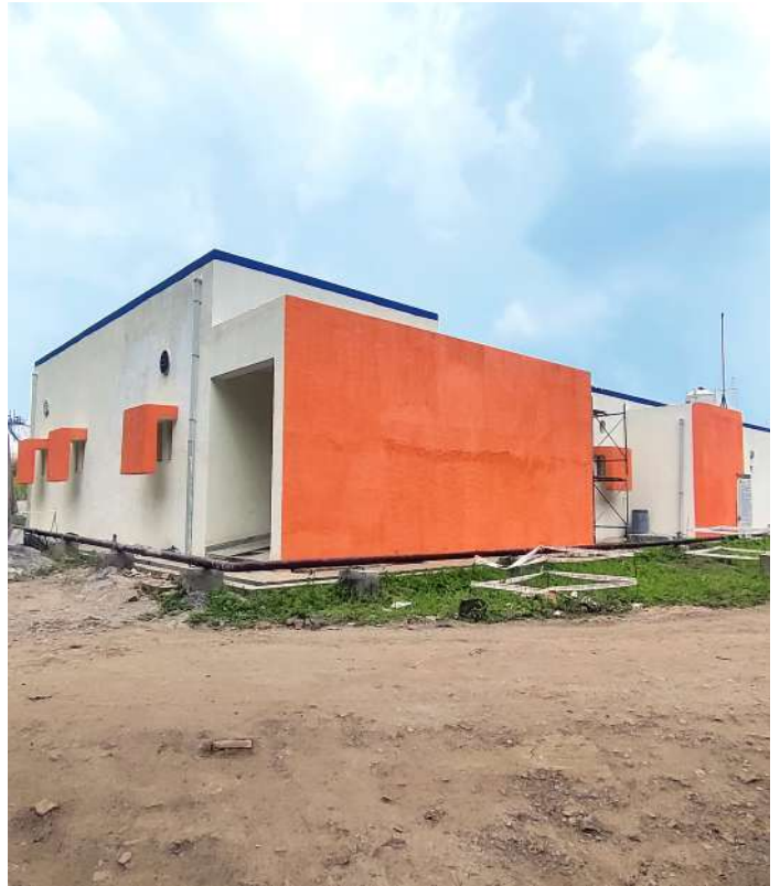
IHB Control Building at IOCL Delivery Station Bhopal ▼
