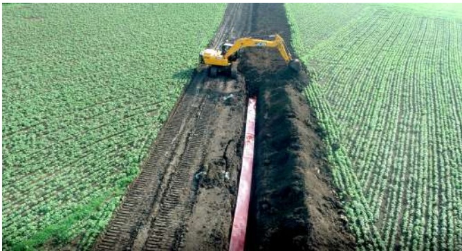
Excavation for Pipeline in MP
