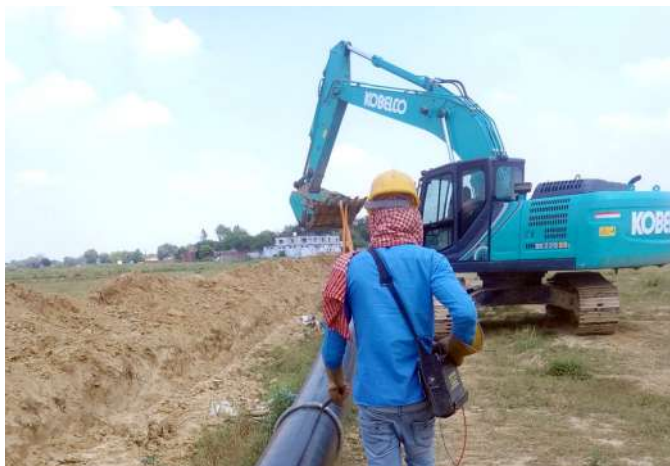
Holiday Testing under progress in UP
