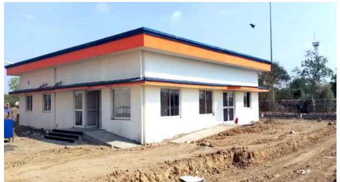
IOCL Sanand Equipment Building
