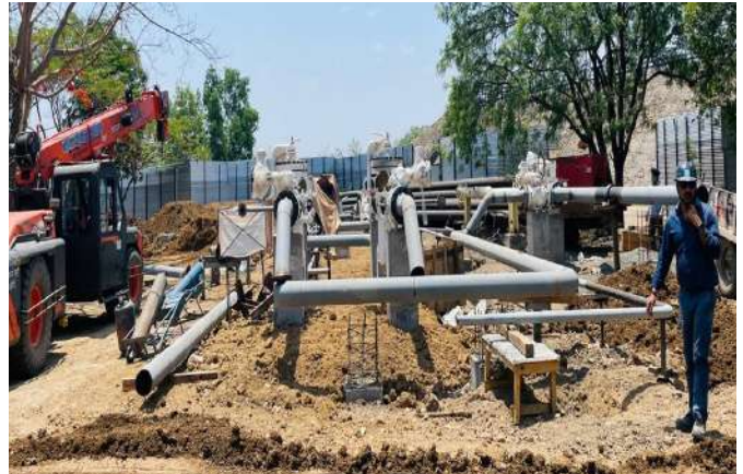
Ongoing station piping work in Indore
